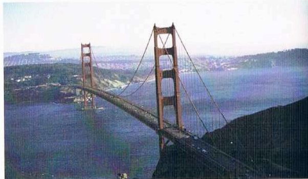
Golden Gate Bridge
