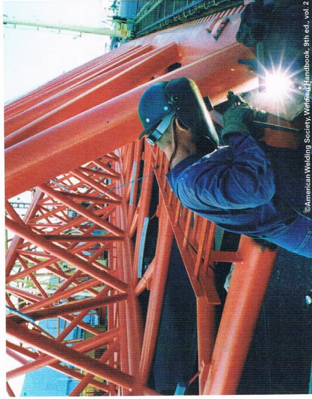
Shielded metal arc welding (or "stick welding")
